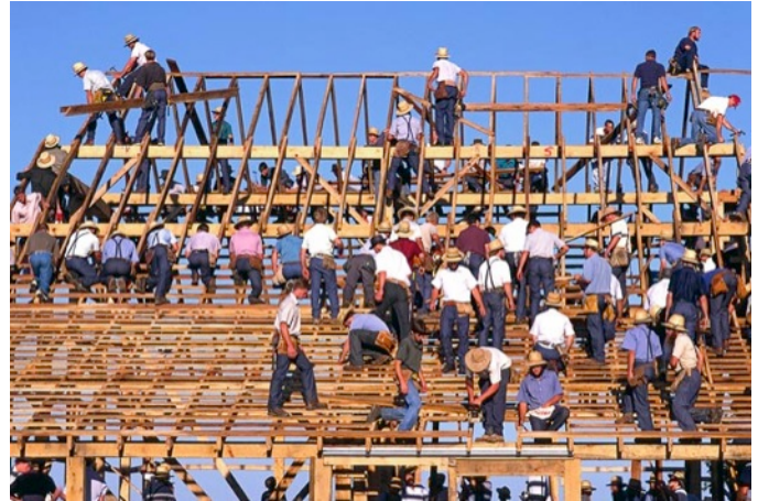
Amish engaged in a barn raising in Lancaster, PA
